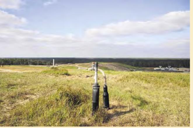
Methane is captured by gas-extraction wells on the landfill surface.
