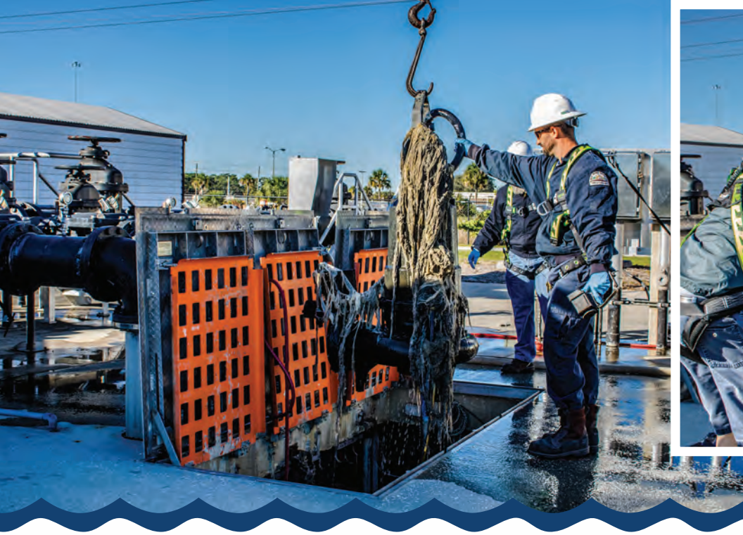
A Hillsborough County Water Resources crew removes a sewer clog caused by people flushing “unflushable” items such as wet wipes down the toilet.
