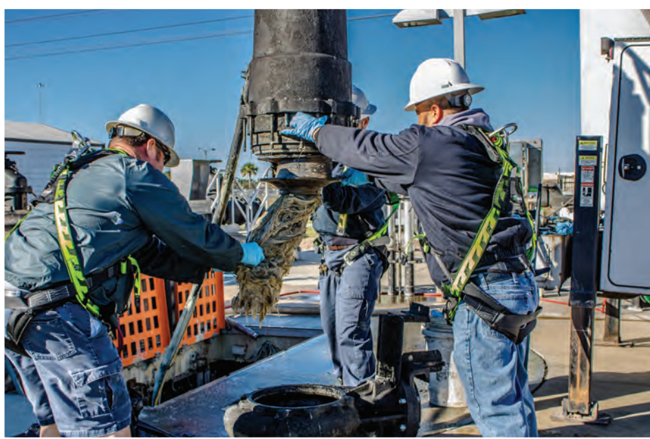
A Hillsborough County Water Resources crew removes a sewer clog caused by people flushing “unflushable” items such as wet wipes down the toilet.
