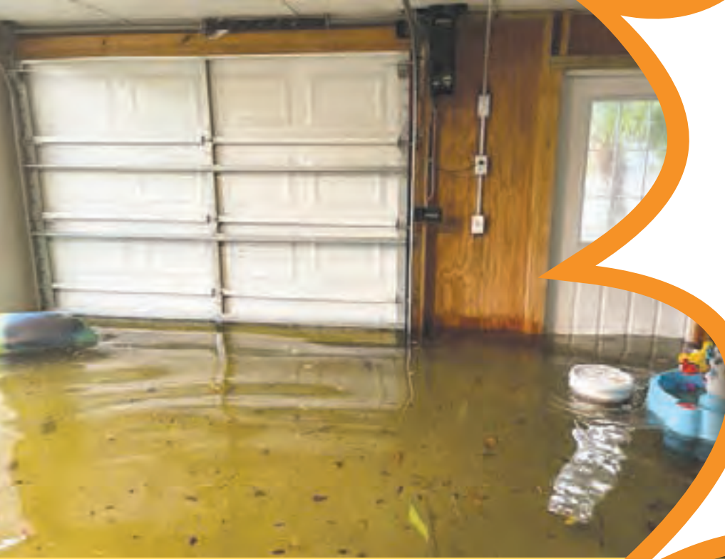
Flooding from Hurricane Idalia in 2023 in St. Petersburg.
