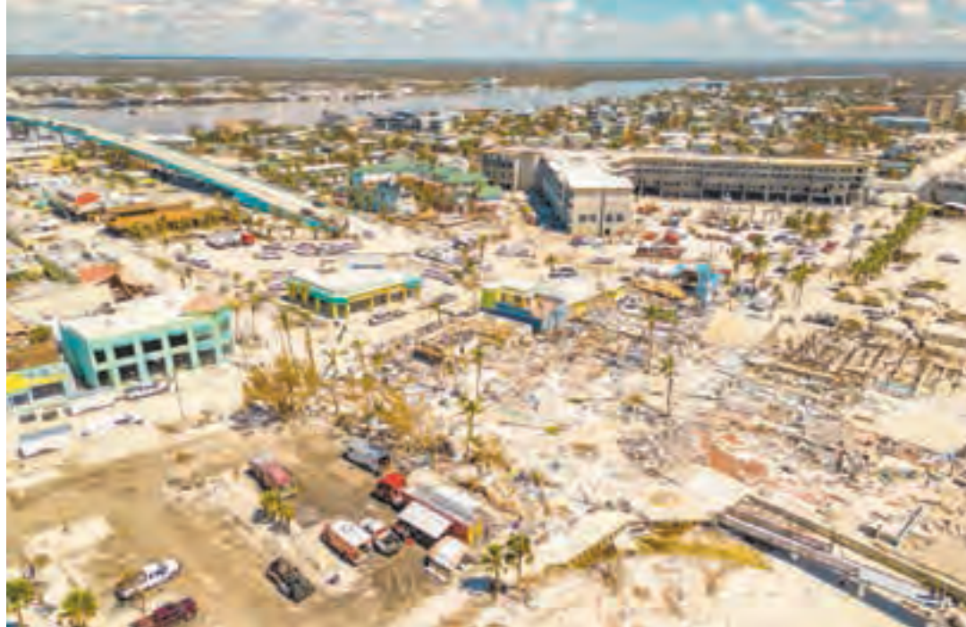
Massive destruction on Fort Myers Beach after Hurricane Ian.
