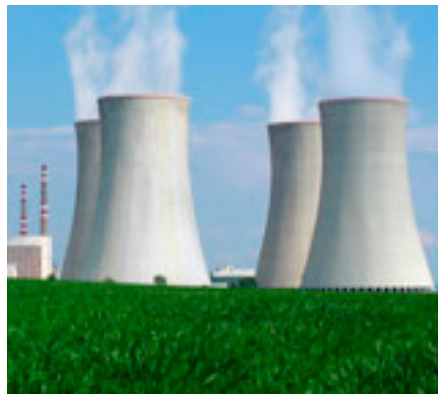
Nuclear cooling towers
