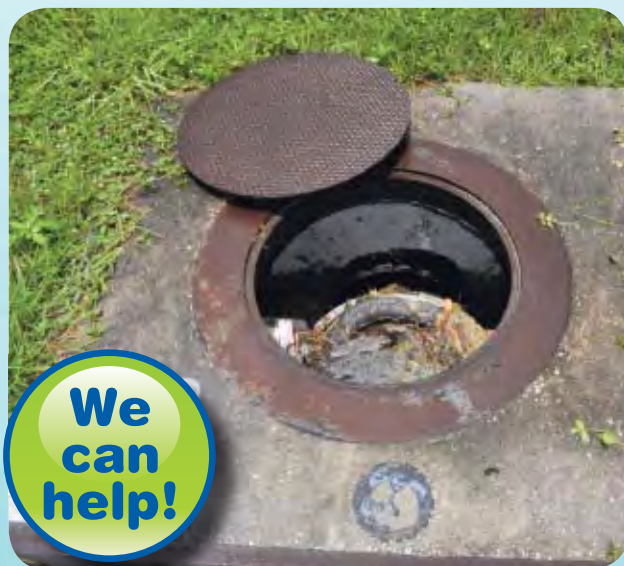
More than 200 of Largo's storm drains have this device to help catch some of the litter and lawn trimmings that would have emptied into waterways. While these baskets help catch some of the debris, we still need your help to keep this stuff out of our stormwater drains!
