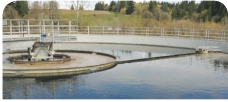
A wastewater treatment tank.
