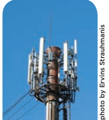
A cellular tower.
