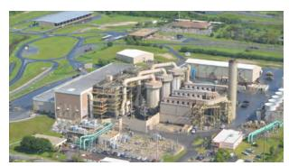
Garbage in Pinellas County is burned as fuel in the County's Waste-to-Energy (WTE) facility. The WTE produces enough electricity to power 45,000 homes each day. The gas produced is cleaned by state-of-the-art air pollution control systems.
