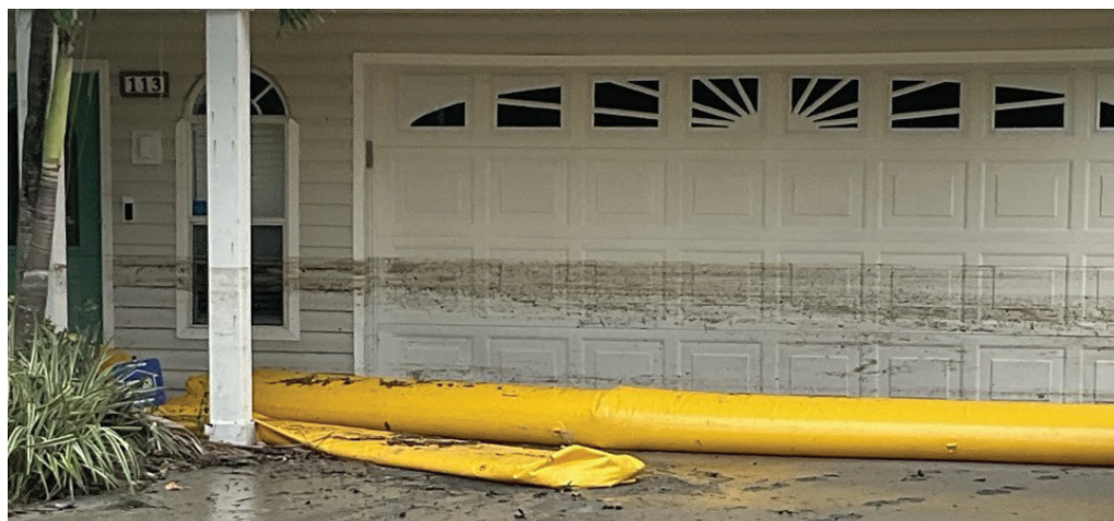
A flood barrier could not protect this home from surge. Times photo
