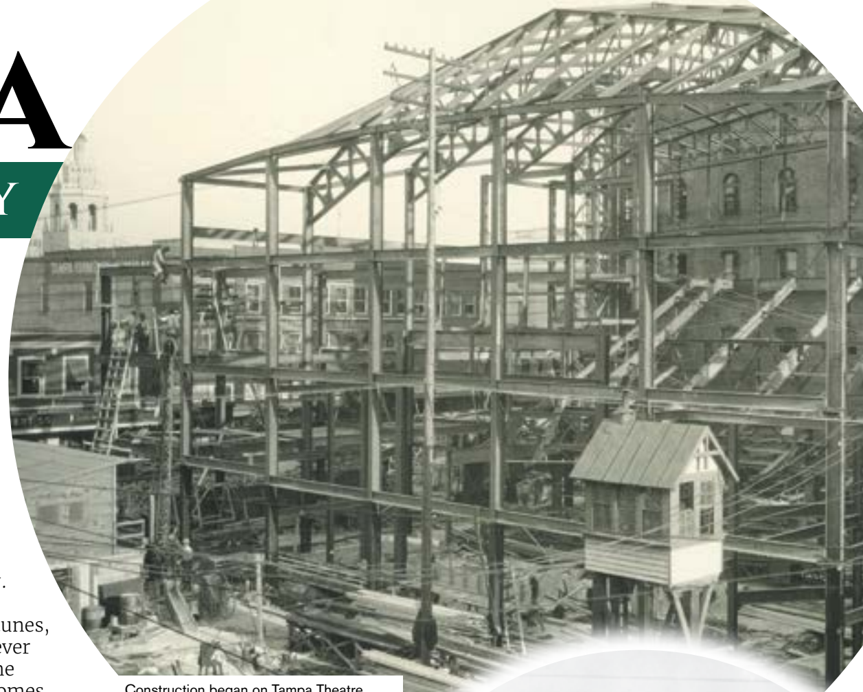
Construction began on Tampa Theatre in late 1925, at the height of the Florida land boom. By March of 1926, the steel structure of the domed night sky was visible above Polk Street. Courtesy of Wolfsonian Archive
